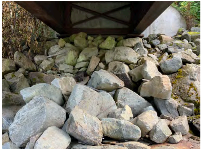
Right Bank Abutment when facing downstream
