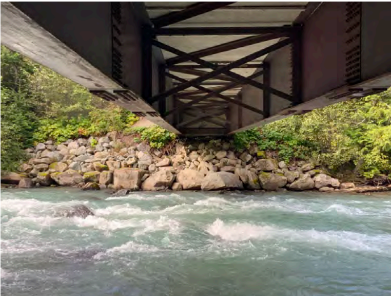
Left Bank Abutment when facing downstream
