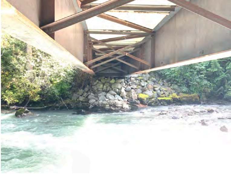
Right Bank Abutment when facing downstream
